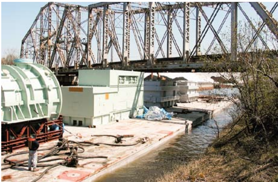
FIG. 3 Special barge can be partially flooded to allow bridge clearance.
