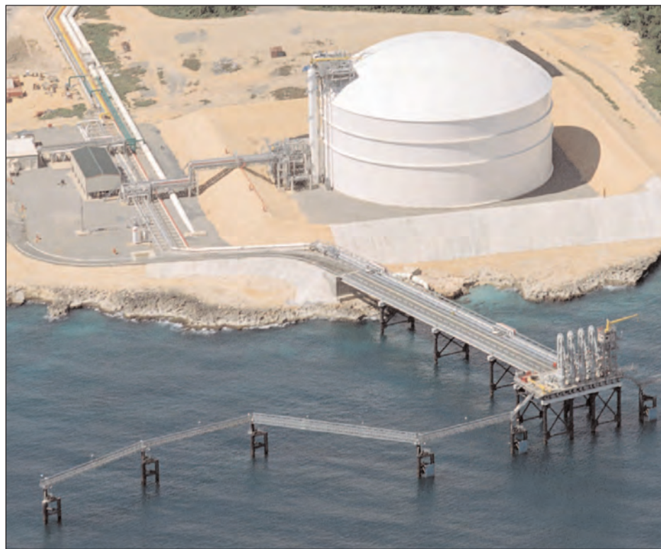
Figure 1: Aerial view of completed AES Andres LNG Import Terminal
