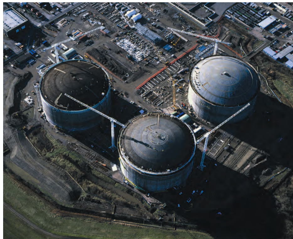
The Isle of Grain LNG facility southeast of London is being expanded to meet higher demand. The US engineering firm CB&I is the main contractor
