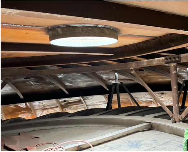
Figure 3. Temporary roof supports.
