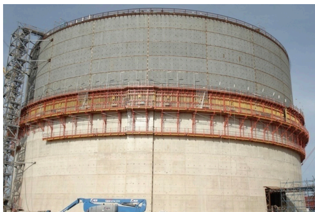
Figure 5. Construction of a full containment tank with free-standing liner.
