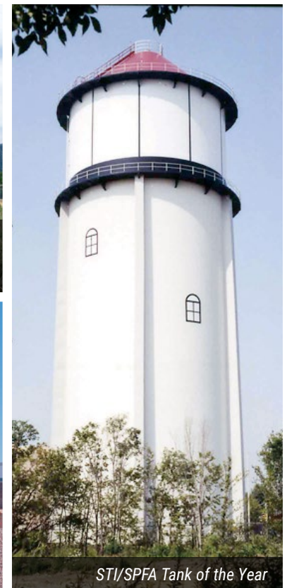
In locations of high visibility, the use of decorative pilasters, special painting, logos or custom shapes can enhance or conceal the appearance of the structure. STI/SPFA Tank of the Year
