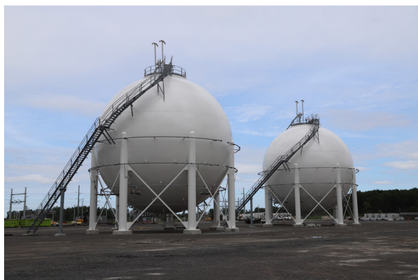
Figure 1. ASME pressure vessel of the year – liquid hydrogen spheres for Plug Power in the US.
