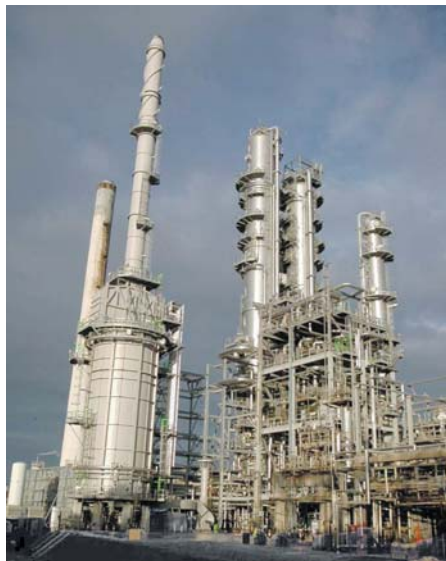
ChevronTexaco CDHydro/CDHDS unit at Pembroke, UK
